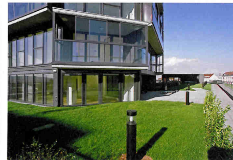
Basis des Elliptenturms Base of elliptic tower
