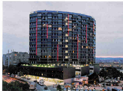
Rote Signalstreifen Neon lines in the facade
